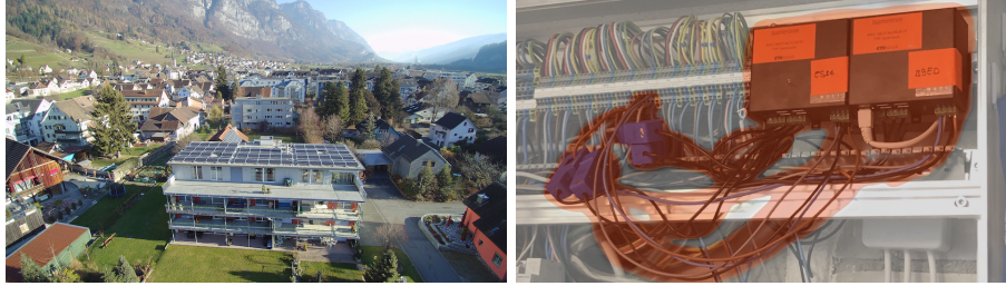
Figure 2: Photos from the Walenstadt microgrid. The left picture shows the large prosumer apartment building with seven apartment units, a 35 kW PV system, and a 23 kWh battery. The right picture shows two SmartPi devices and attached current transformers (in red) installed in a circuit breaker box in a single family prosumer building.
